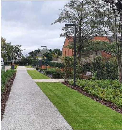
Fig 9 - Exposed aggregate concrete footpaths
