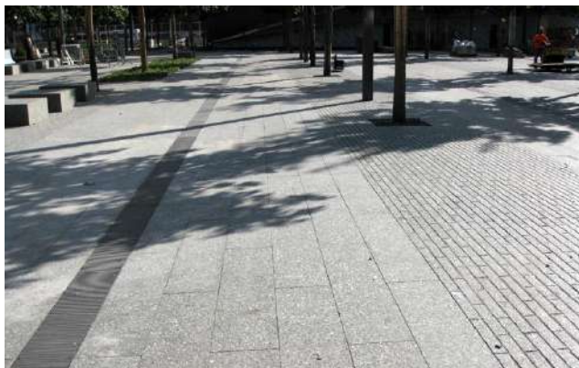
Fig 12 - Stone Paving, Silver Granite Slabs, Flamed finish
